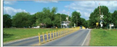
Gates with Channelization Devices
